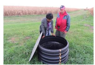
George Cummings showing us a denitrification plant at the experimental farm. This plant prevents accumulation of nitrates in ground water due to fertilizer use
