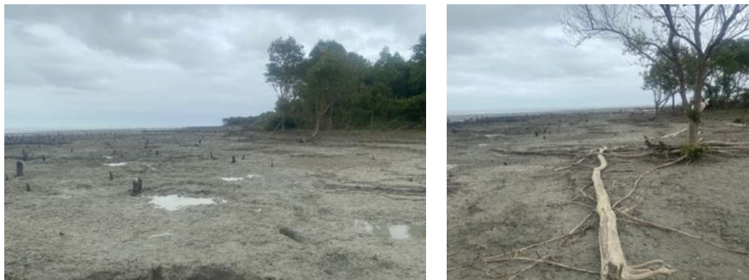
Figure 7: Coastal damage to Kondo Village due to sea waves
